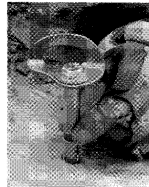
Placing A Bolt With Hanger Into Finished Hole
