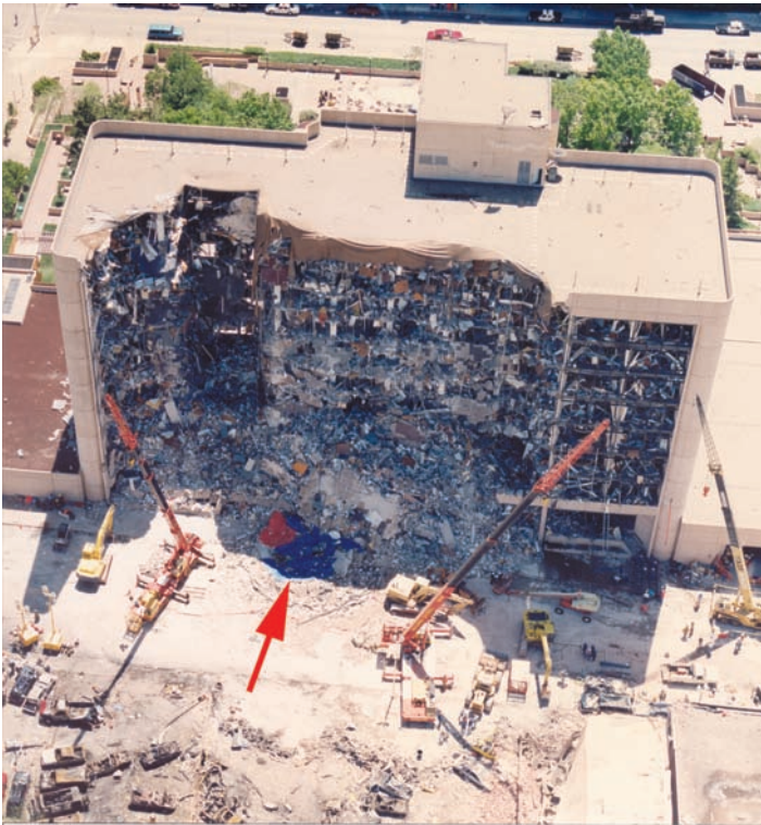
Figure 14.1. An aerial view showing the damage to the Alfred P. Murrah Federal Building. The Ryder truck bomb had been parked in front of the building. A crater was now at this location and is covered by blue tarp, as indicated by the arrow.
